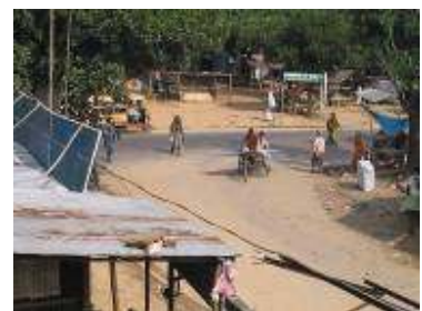
Fig.5: Uncontrolled and poorly designed access road
