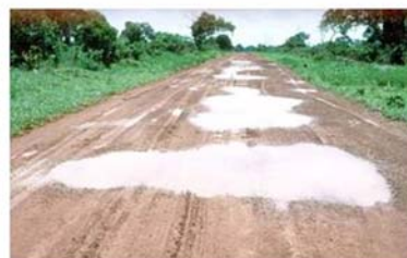
Figure 3 - Maintenance of gravel roads
