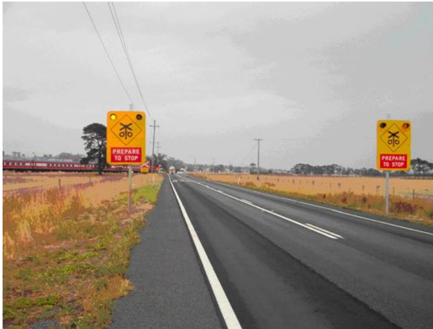
Figure 4 – Automated advance warning signs
