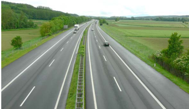
Figure 2 – Measurement location on the A2-Highway [5]
