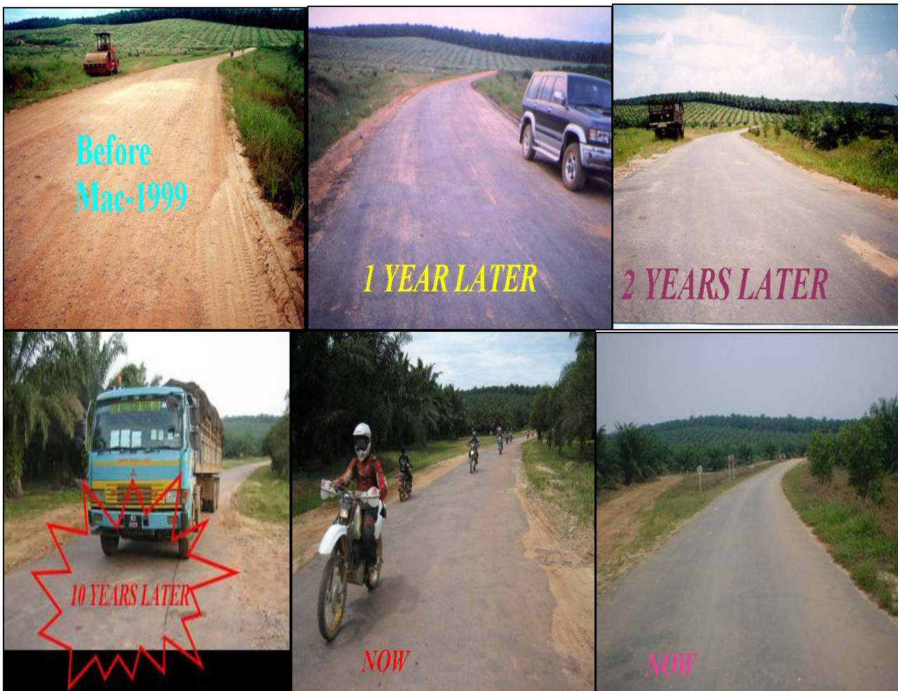
Figure 16 – The performance of soil stabilization road
