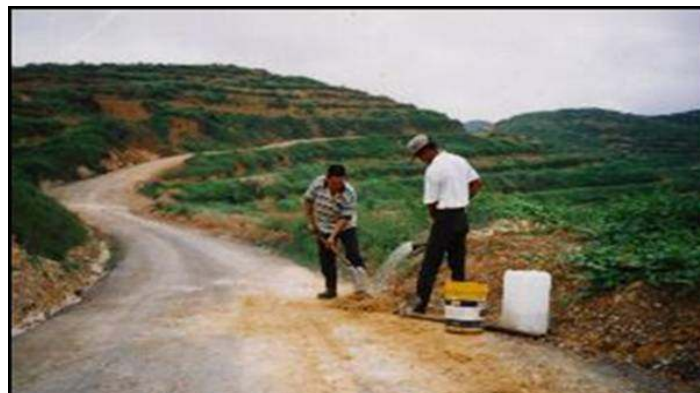
Figure 12 – Mixing soil with soil stabilizer agent
