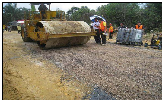
Figure 10 – Spreading the chipping stone
