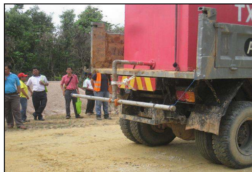
Figure 7 – Spraying the soil stabilization agent
