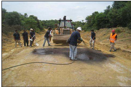
Figure 9- spraying the waterproof sealant on the road surface
