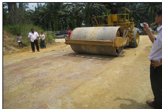
Figure 8 – Compaction work using roller compacted 10tonne
