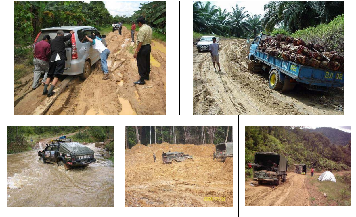
Figure 3 – Overview of the Rural Road
