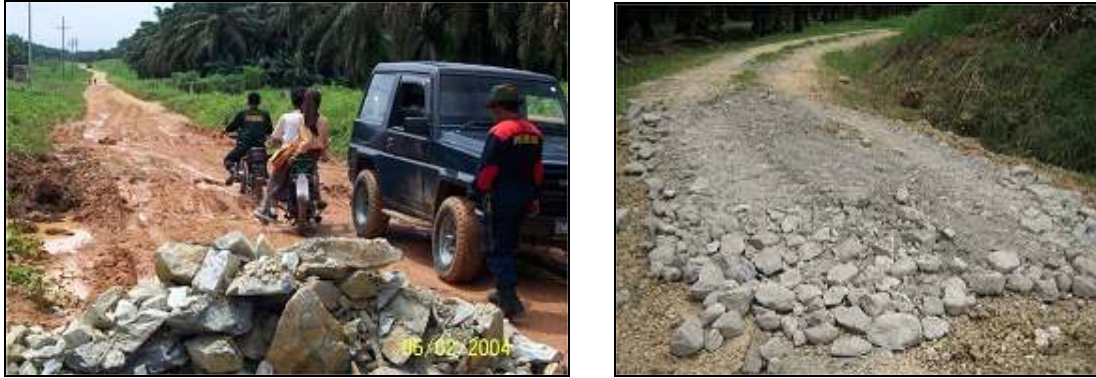
Figure 14 – Patching works using stone for conventional method
