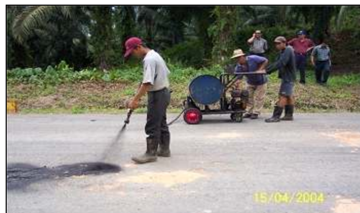
Figure 13 – Applied the sealant on the road surface
