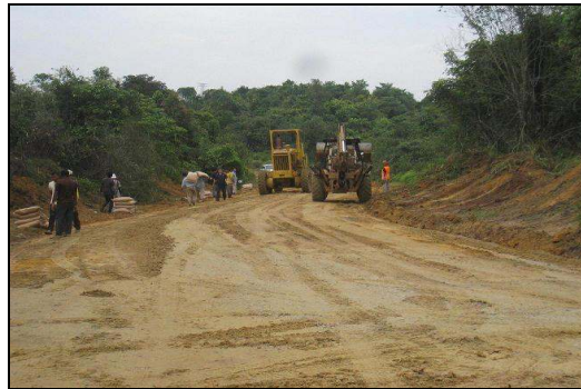
Figure 6 – Loosening existing soil
