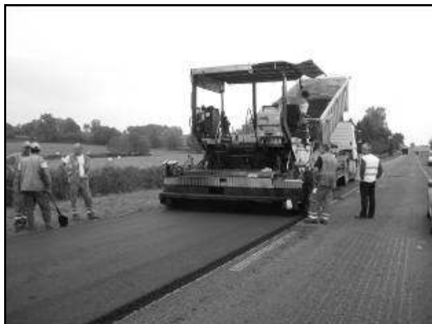
Photo 3 – Roadworks 2009 RD 981 CG 58
