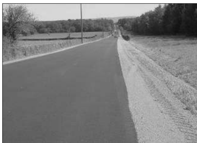
Photo 4 – Roadworks 2007 RD 978 CG 71
