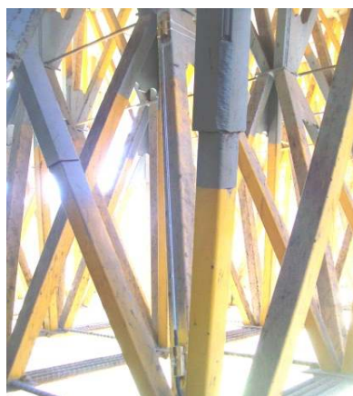
Figure 4 – Installation of optical strands on tubular profiles
