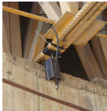
Figure 3 - Optical strain gauge on supports; detail
