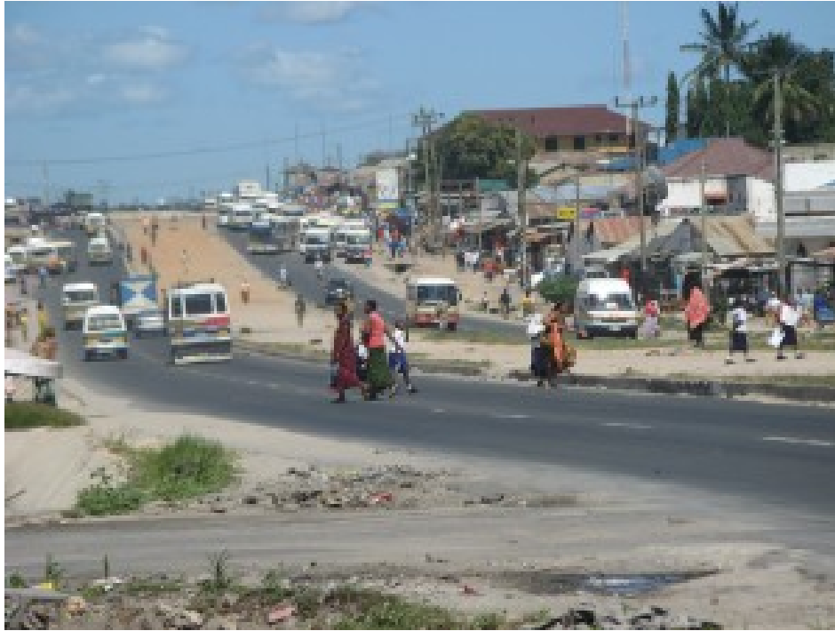
Figure 1 - Tanzanian roads bearing mixed traffic, unshouldered pedestrian crossing, markets and dwellings 10
