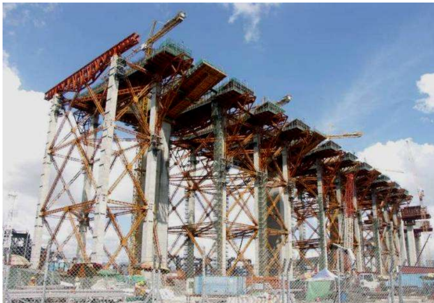
Figure 7 – Back Spans under Construction
