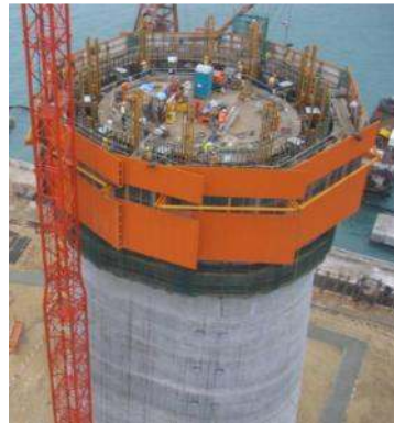
Figure 10 - Lower Tower Construction
