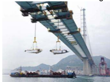
Figure 14 – Main Span Closure
