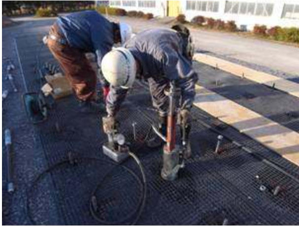
Photograph 7 - Anchor locking
