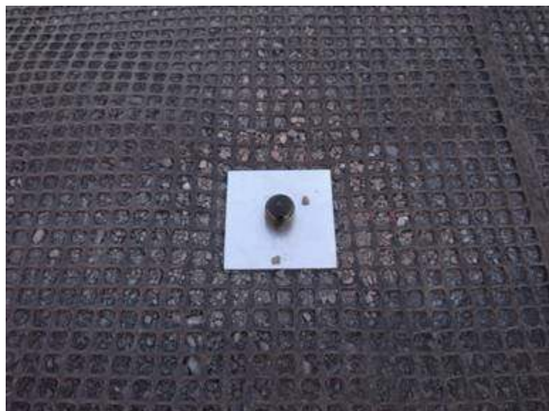
Photograph 10 - Top of the anchor
