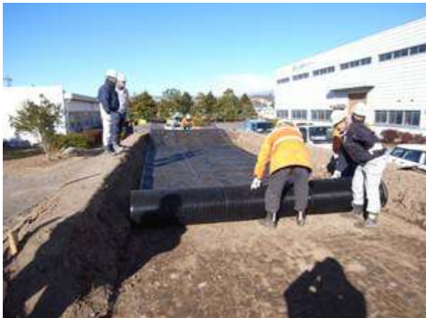
Photograph 3 - Geosynthetics placement
