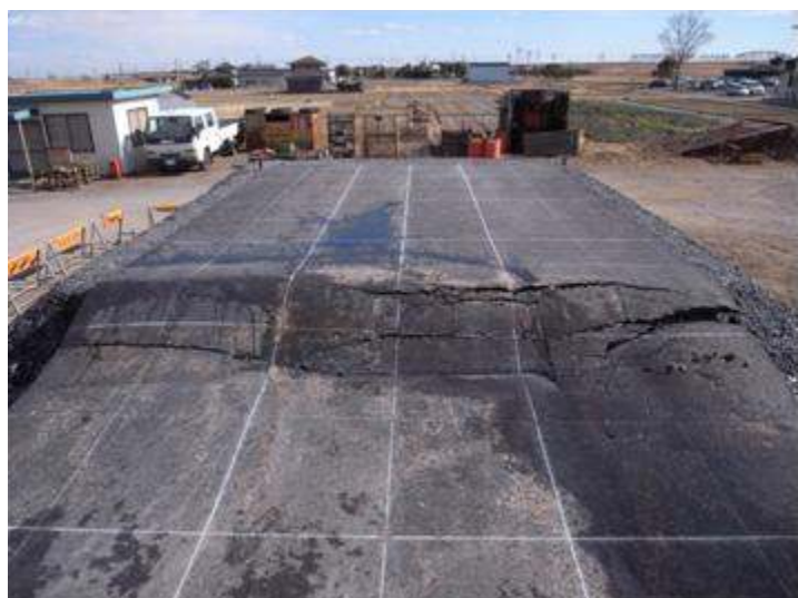
Photograph 14 - Deformation of asphalt pavement on normal pavement after 300mm forced settlement
