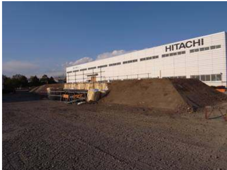
Photograph 12 - Trial embankment
