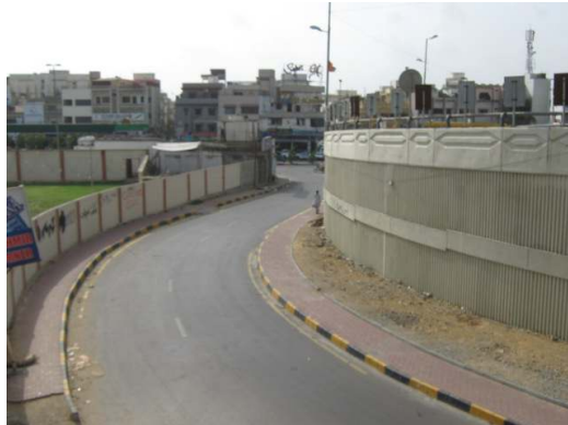
“Figure 6 - Absence of Ladder and Manned Zebra crossings at sharp bends”
