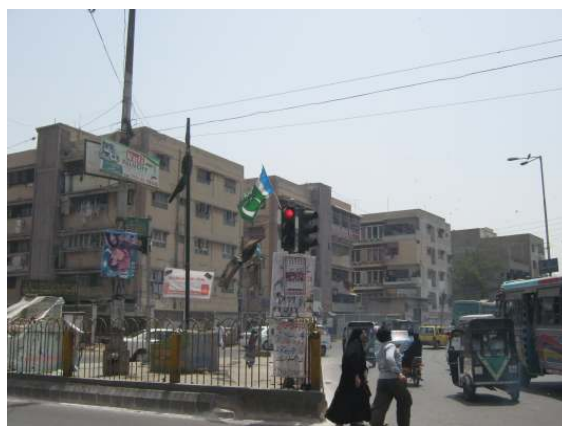
“Figure 9 - At Grade Crossing with the provision of Fencing at Signalized Staggered Intersection”
