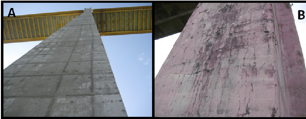
Figure 2 photographs A) pile 4 Mezcala and B) pile 5 Dovali
