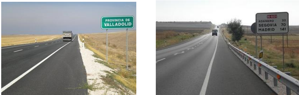
Figure 6 – Examples of absence and presence of Safety barrier on the N601
