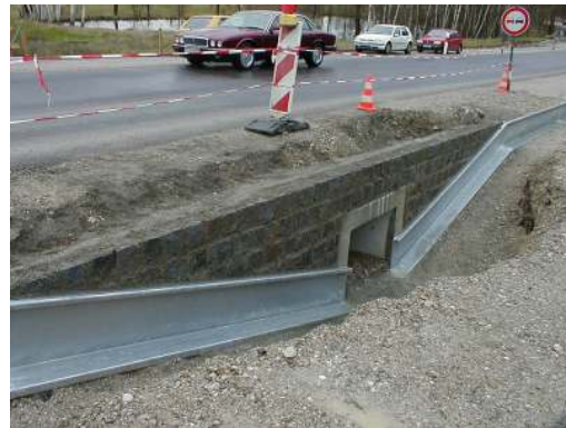
Fig. 4 – Amphibian Crossing Culvert and Guiding Guardrail, designing detail and construction solution [8]
