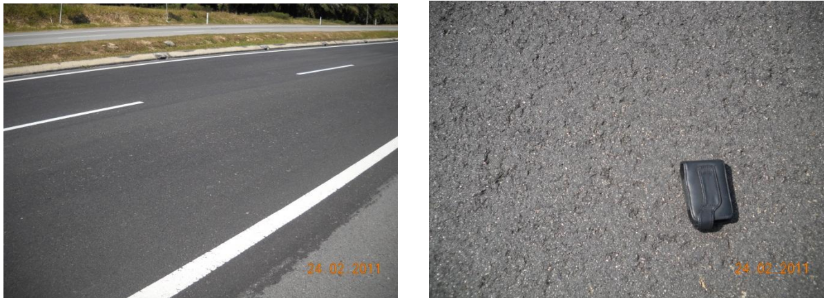
Figure 7 - Pavement surface at the HIPR without addition of rejuvenating agent
