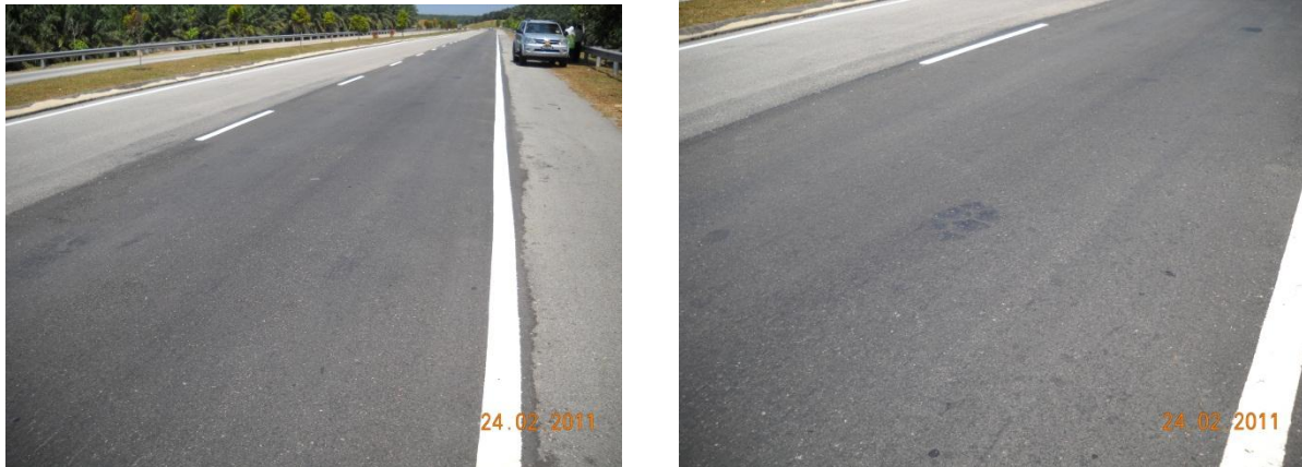
Figure 9 - Apparent bleeding at the HIPR with addition of 0.5% rejuvenating agent
