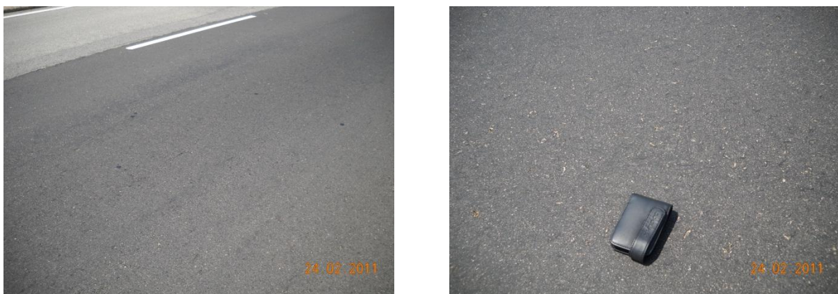
Figure 8 - Bleeding at the HIPR with addition of 0.3% rejuvenating agent
