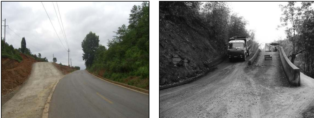
Figure 10 - Original overload disposal
