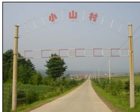
Figure 8 - Breakaway height restriction barriers
