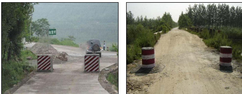
Figure 3 -Width restriction blocks of village road
