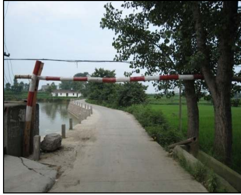
Figure 9 - Height restriction barriers raised and lowered
