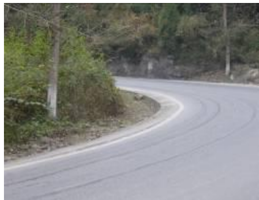
Figure 2 - Poor sight distance
