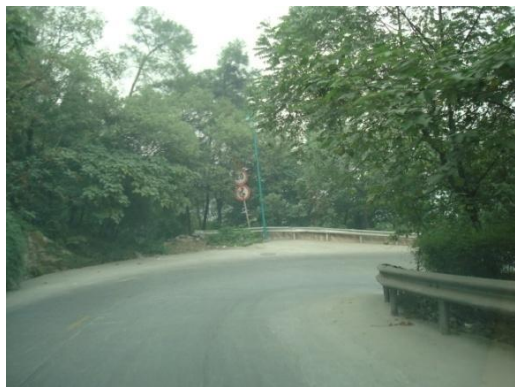
Figure3 - Continuous curve and poor sight distance
