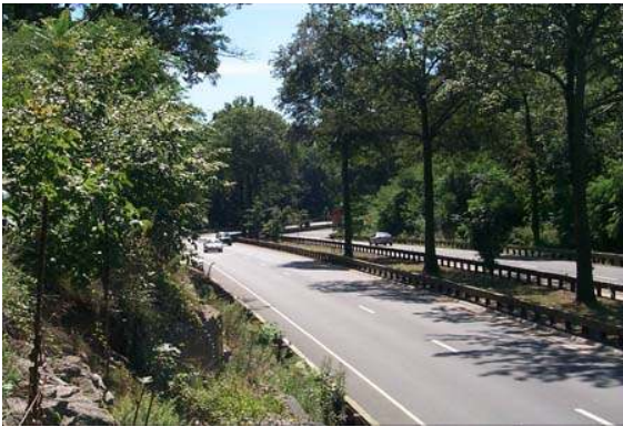
Completed Merritt Parkway Section
