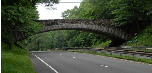
Guinea Road Bridge - Stamford
