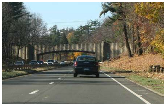
Madison Road Bridge During Construction
