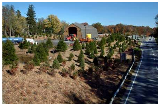
Newly Constructed Salt Shed
