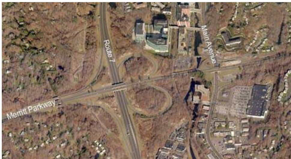
Route 7 /Route 15 Interchange
