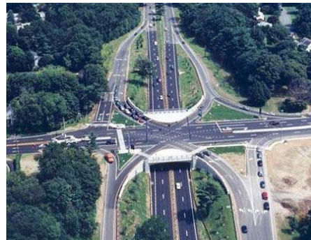
Aerial View of Single Point Interchange
