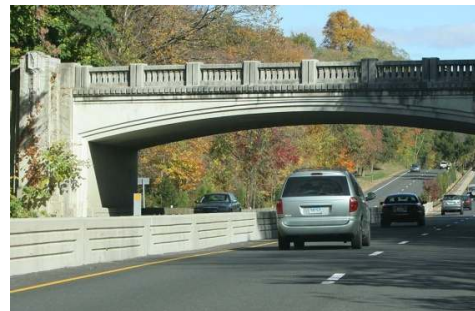
Merritt Parkway Concrete Barrier
