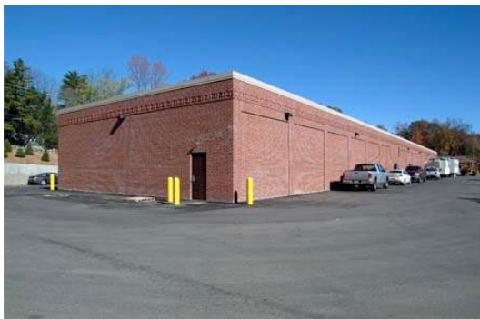
Newly Constructed Maintenance Building
