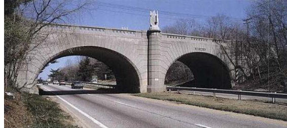
James Farm Road Bridge - Stratford
