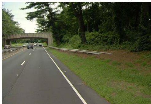
Madison Road Bridge Prior to Construction
