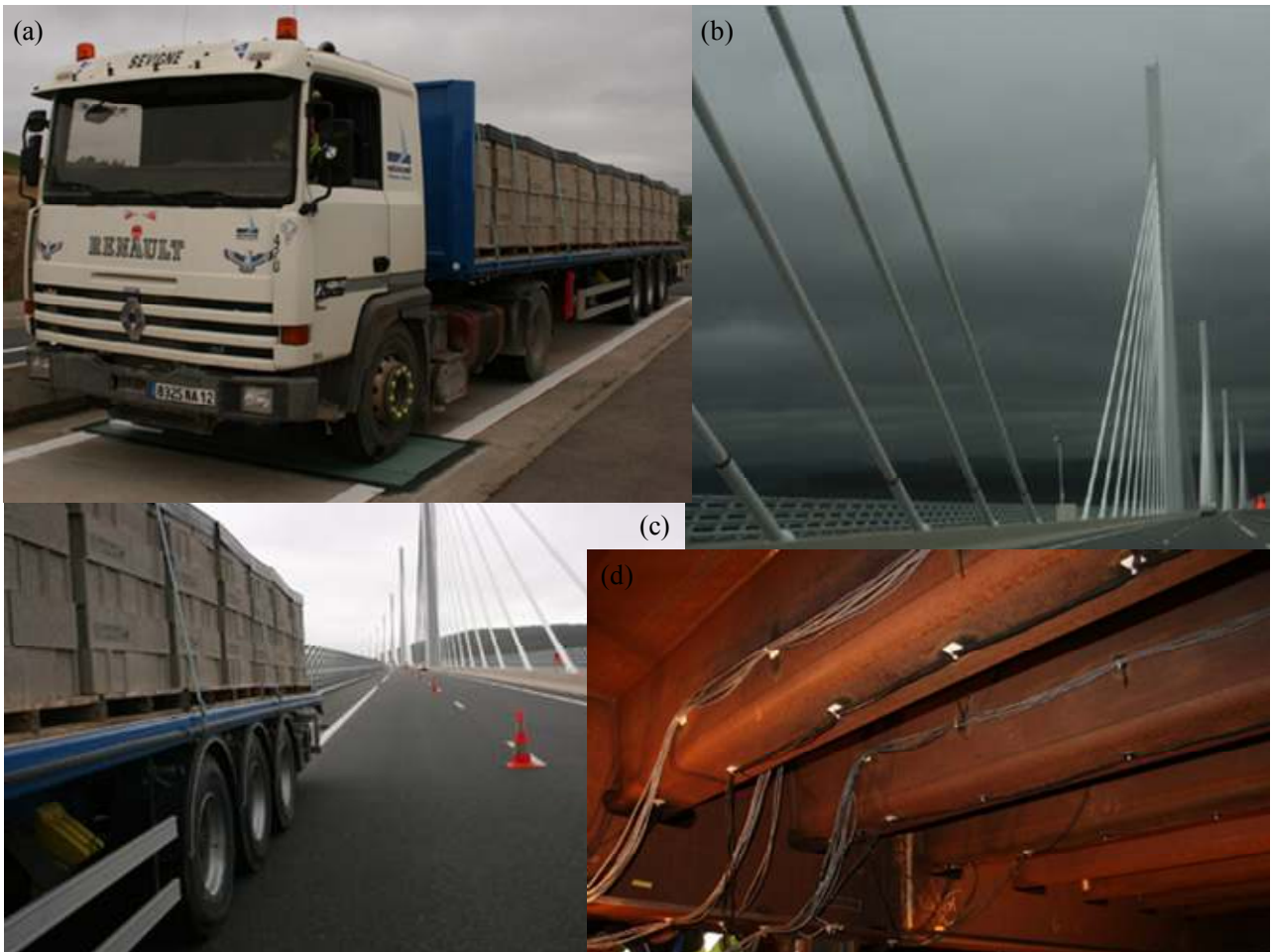
Figure 8 – Pictures of the Millau Viaduct during tests. (a) Truck during axles weight; (b) View of the bridge; (c) Loading truck on the Millau Viaduct; (d) Stiffeners and crossbeams with gauges
