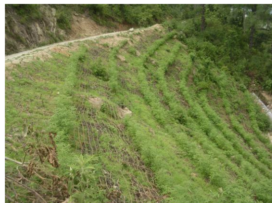
Figure 2 - Same site after bio-engineering combination of jute netting, brush layering and grass seeding
