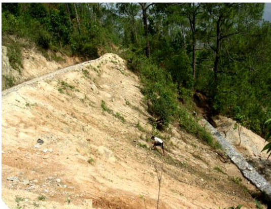
Figure 2 - Same site after bio-engineering combination of jute netting, brush layering and grass seeding
