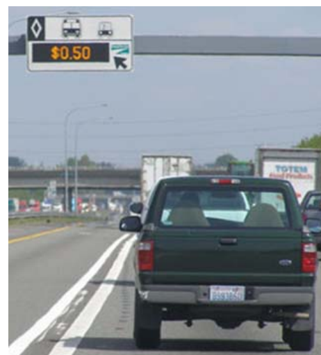
Figure 4: Dynamically tolled HOT lane SR 167
