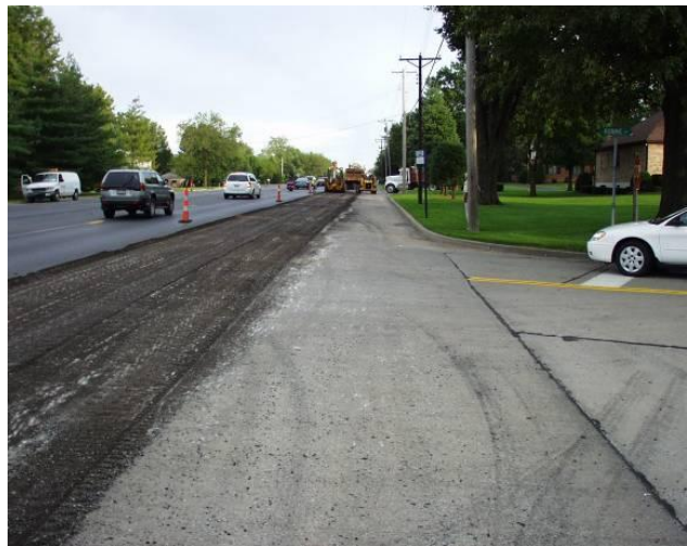
Lindbergh - During Construction
