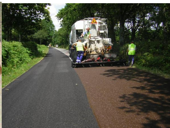
Picture 2 - Laying of the microsurfacing
