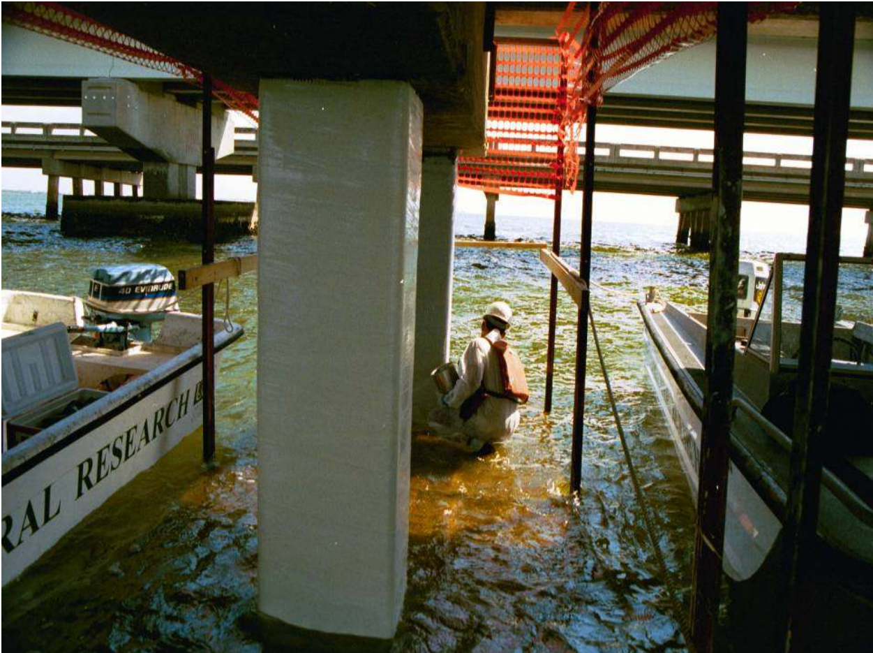
Fig. 3 FRP repair of corroding pile, Tampa Bay, FL
