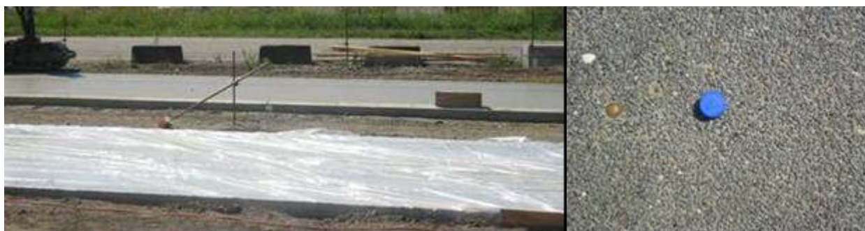
Figure 11 – Trial section of double layered concrete with \text{TiO}_2 on the top layer in industrial zone “Den Hoek 3” in Wijnegem
