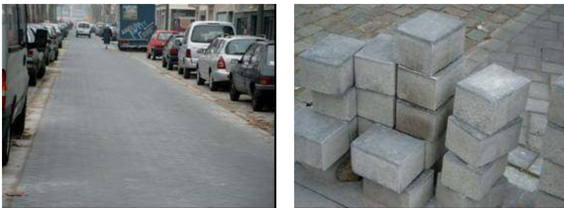
Figure 5 - Separate parking lanes at the Leien of Antwerp with photocatalytic pavement blocks.
