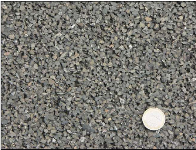
Figure 3. Example of a surface of a proprietary thin asphalt layer called “Microflex” paved on Kasteelenlaan in the Dutch city of Ede; four years old here; aggregate size 2-6 mm. Paved primarily due to its noise-reducing capability. Note that chippings have a flat surface facing upwards.
