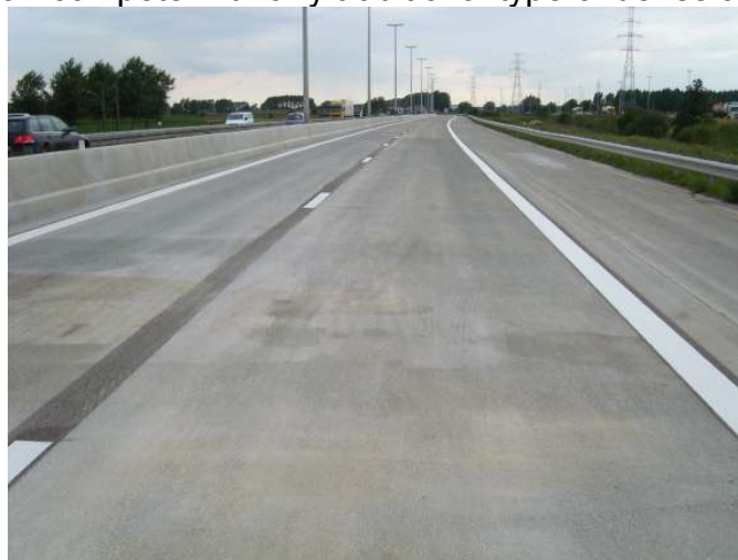
Figure 7 – the finished pavement and barrier
