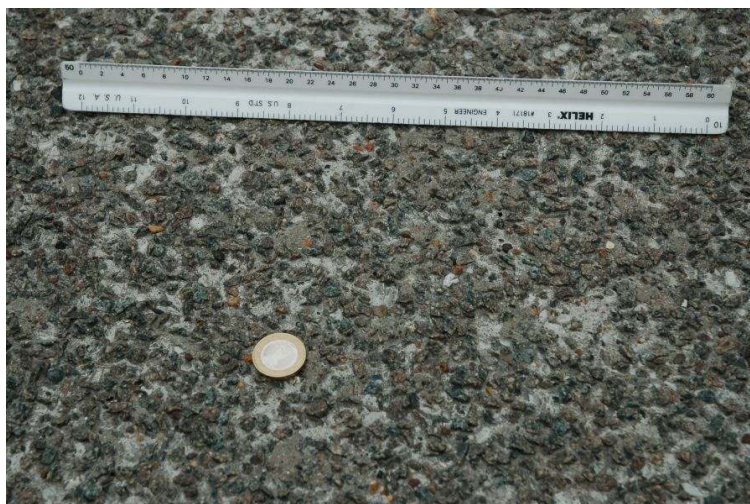
Figure 6 – the exposed aggregate concrete surface
