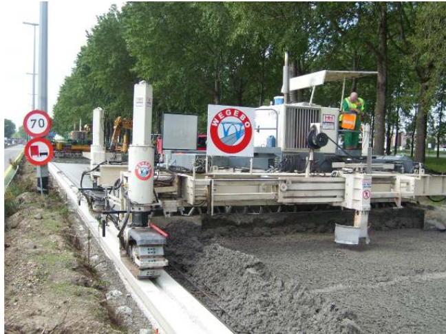
Figure 5 – worksite in progress by two slipform pavers
