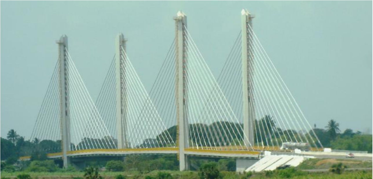
Figure1 – General view of the Rio Papaloapan Bridge
