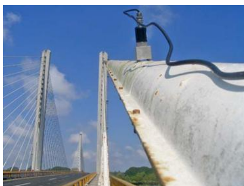
Figure 14 - Typical accelerometer location for the vibration measurements
