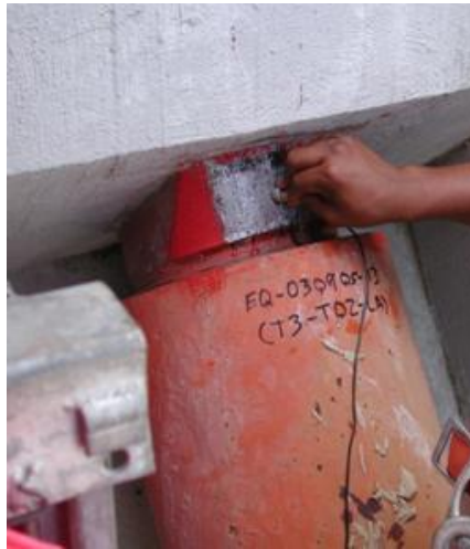
Figure 10 - Accessibility for the ultrasonic inspection of a cable upper anchorage element
