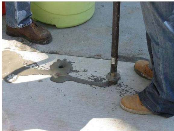
FIGURE 9 JPPS installation on connector ramp (from top left: precast panel fabrication, removal of existing pavement for recycling, grading of base, panel installation, grouting of dowel slots/underslab, and installed panels next to existing left lane).
