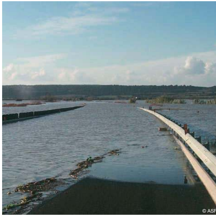
Figure 1 - 04 December 2003, inundation of the Rhône river valley in South of France. The A54 motorway was flooded during 11 days.
