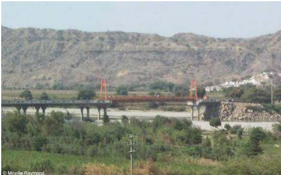
Figure 3 - Large bridge destroyed by an El-Niño episode in 1998
