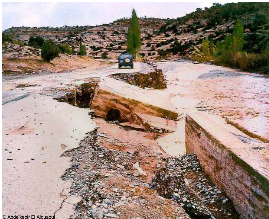
Figure 2 - Destruction of a provincial road by a flash flood in the Atlas Mountains (Morocco, 2006)
