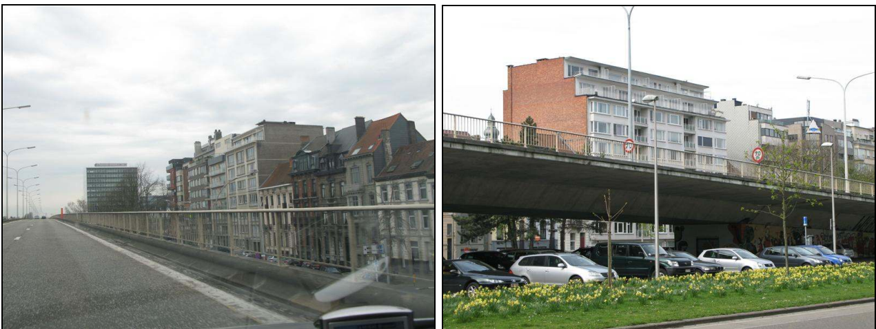
Figure 2 – Typical high-speed road in Gent (Belgium) causing severe noise nuisance at the surrounding dwellings and for which PERS would be an excellent solution.
