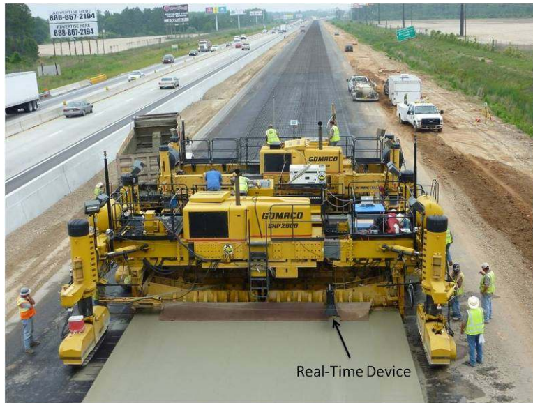
Figure 6 - Real-time smoothness measuring device attached to the concrete paver.
