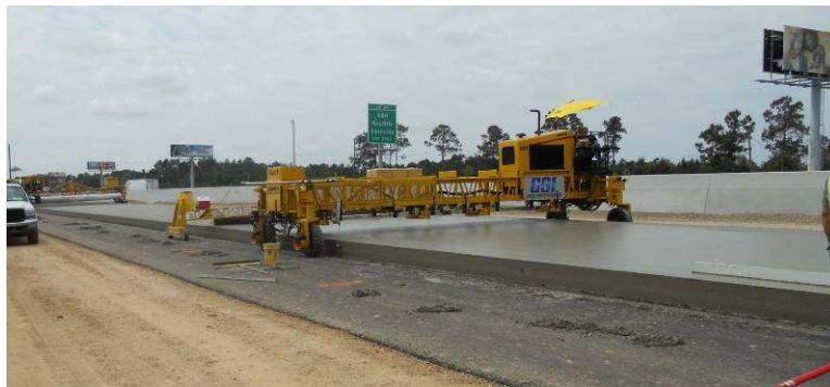
Figure 7 - Stand-alone real-time smoothness measuring system.
