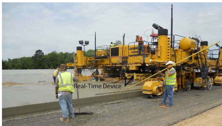
Figure 8 - Real-time smoothness measuring device attached to the concrete paver.
