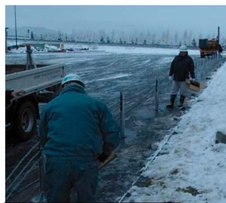
Photo16(right) Wire rope trial installation (NEXCO East Asahikawa)
