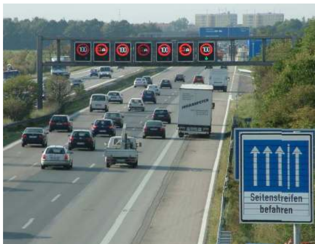
Figure 1 - 3-lane plus shoulder opened with Variable Message Signs near Munich, Germany
