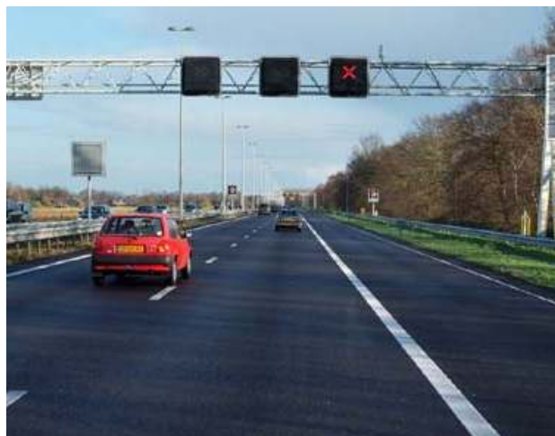
Figure 2 - 2-lane plus shoulder closed in the Netherlands; Source: Rijkswaterstaat
