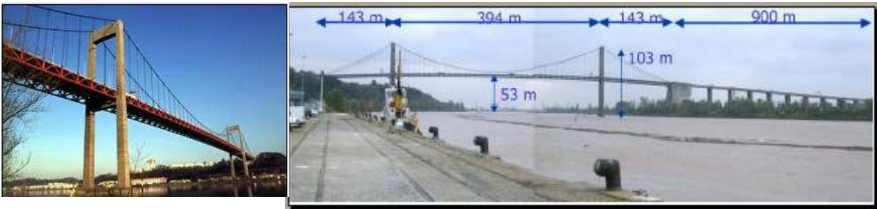
Figure 1- Characteristics of the original bridge -Source SETRA
