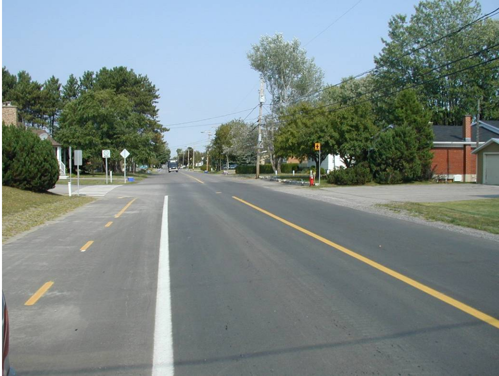
Photo 2 – Saint-Louis de France – typical road after maintenance work
