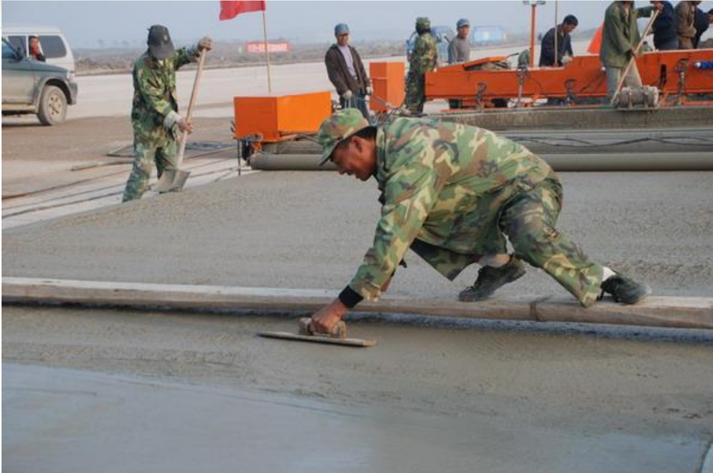
Concrete finishing
