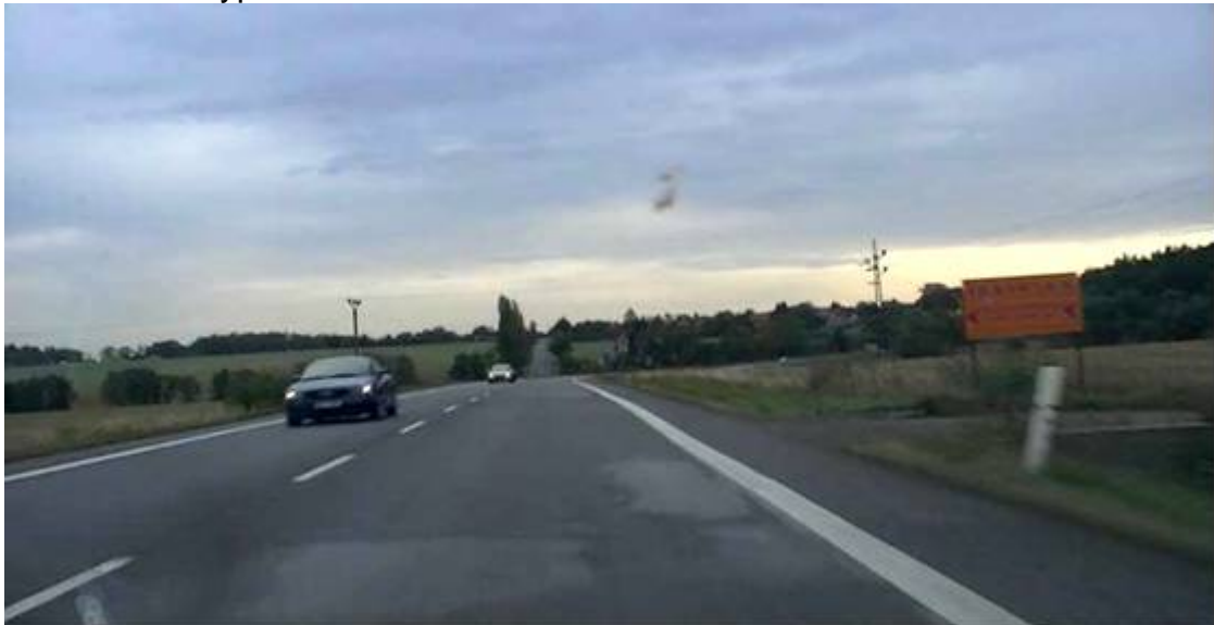
Figure 11: Confusing road alignment – road actually turning to the right to by-pass, straight on old road scheme. Overtaking is very hazardous.
