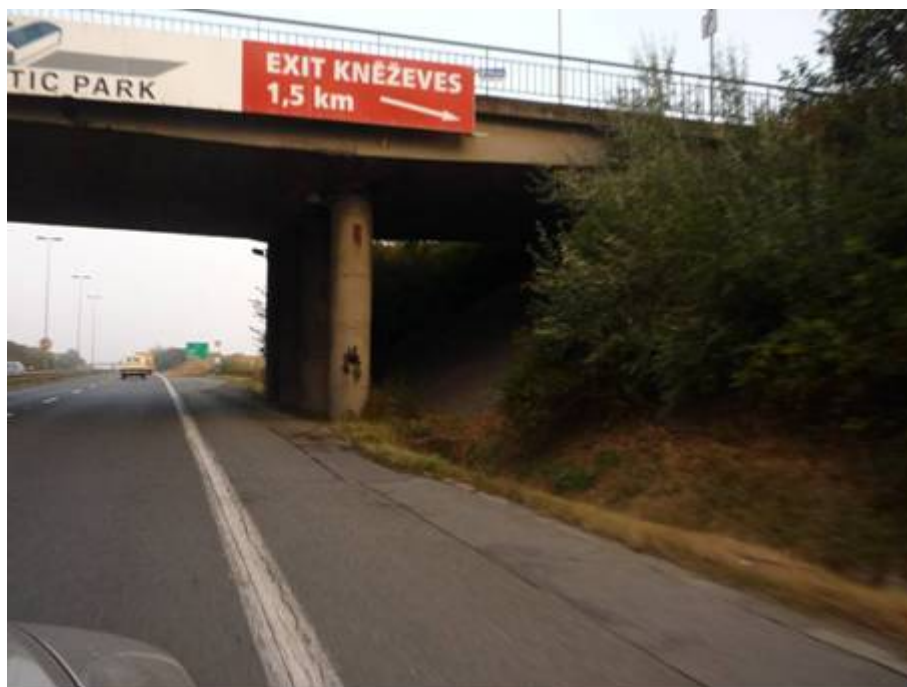
Figure 15: Two lives lost in two accidents at the older motorway not equipped with guard rails at the bridge columns
