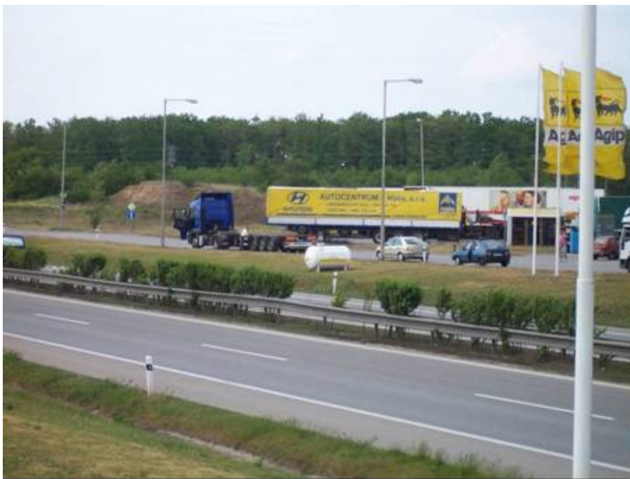
Figure 17: Gas tank close to motorway traffic lanes (D8)
