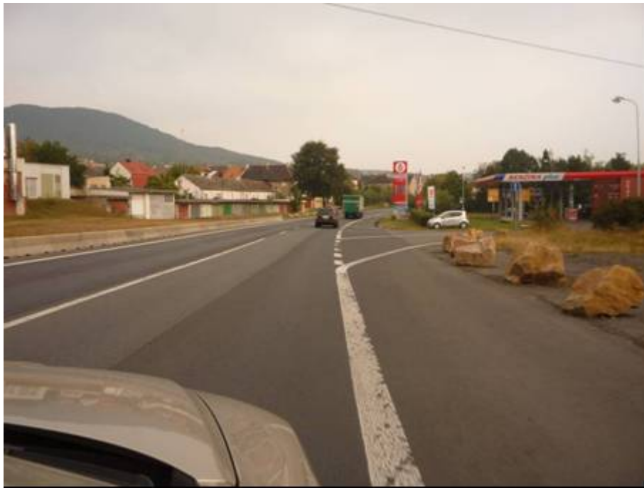
Figure 16: First class road (I/30) of European importance equipped by boulders instead of delineators.
