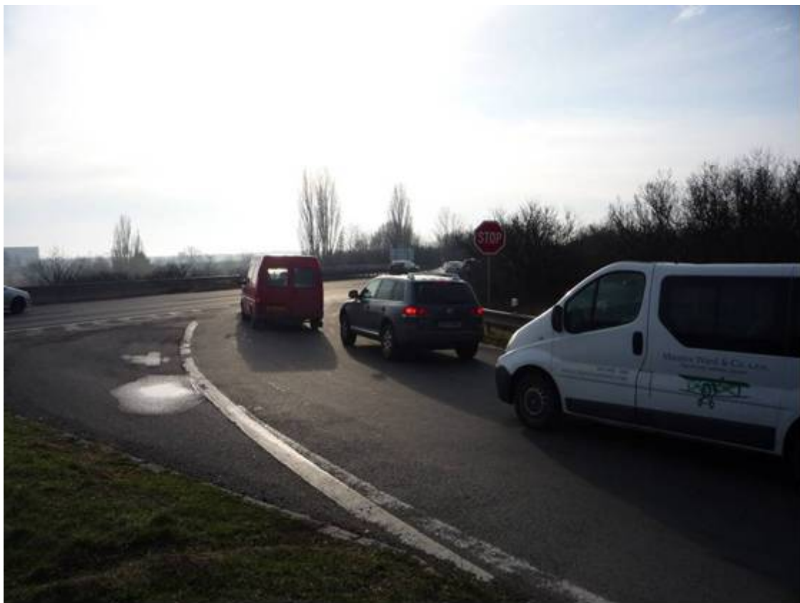
Figure 13: Expressway interchange without acceleration lane
