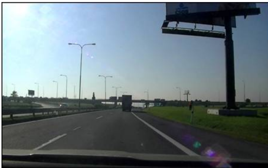
Figure 19: Advertisement "Mega-board" structure close to motorway round Prague (SOKP 516)
