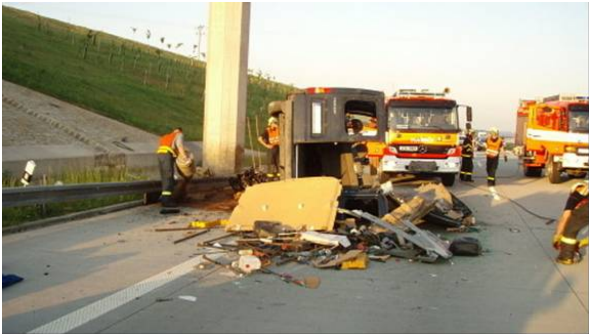
Figure 14: Tragic accident on the newly opened motorway D47 – impact to bridge pier
