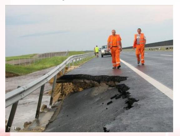
Extreme rainfall  $\rightarrow$ too much water into improperly compacted shoulder of M6  $\rightarrow$  erosion of hard shoulder and slope  $\rightarrow$  traffic restriction for 1 week
