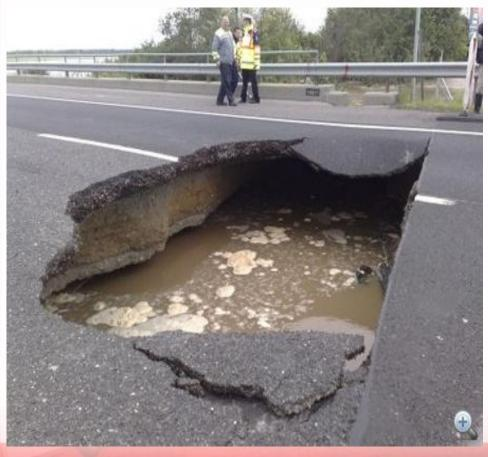
Extreme rainfall  $\rightarrow$  too much water to culvert under M1  $\rightarrow$ erosion  $\rightarrow$  caving-in of pavement structure  $\rightarrow$ traffic closure for 4 days
