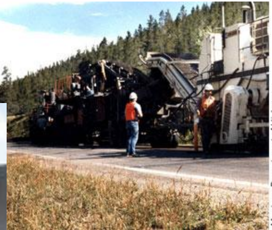
Montana Department of Highways
