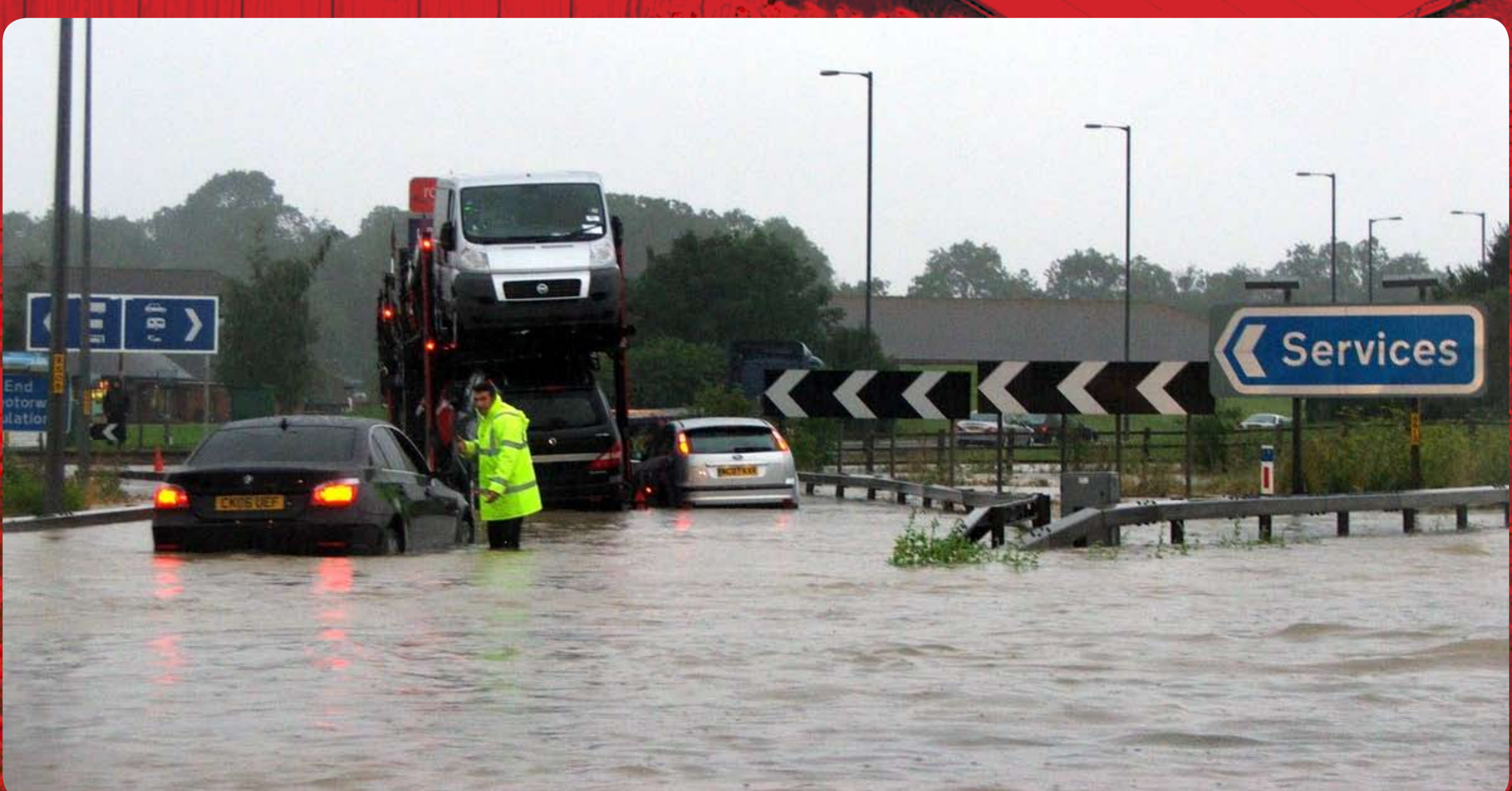
Climate change adaptation is essential for transport authorities (Strensham flood UK: The motorway running near to the services was completely cut off in two locations during the July 2007 floods.)
