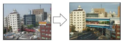
Before elevated railway bridge After elevated railway bridge Figure 4.1.4 - Measures for bottleneck railroad crossings (Keikyu Main Line/Airport Line grade separation project)
