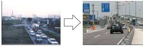
Before intersection grade separation After intersection grade separation Figure 4.1.3 - Grade separation project of intersection (Ordinary National Highway 17, Kakinuma-Koizuka grading [Kumagaya, Saitama])
